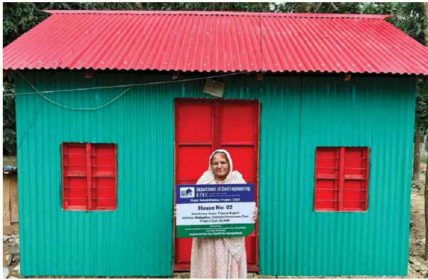
New home for a flood-affected family in Mali Pathor, Parshuram
